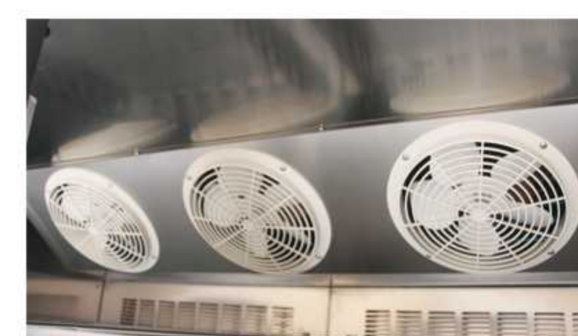
3-fan-assisted evaporator
