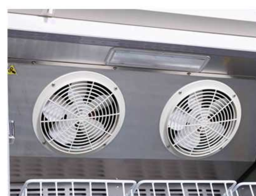
2-fan-assisted evaporator
