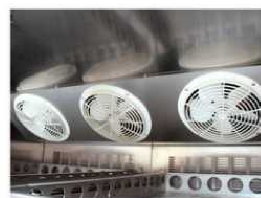
3-fan-assisted evaporator
